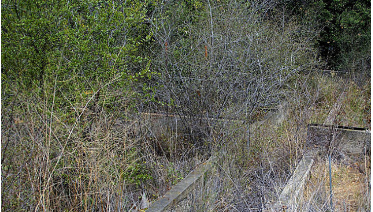
A portion of the over-grown foundation of what was once a state-of-the-art greenhouse.
